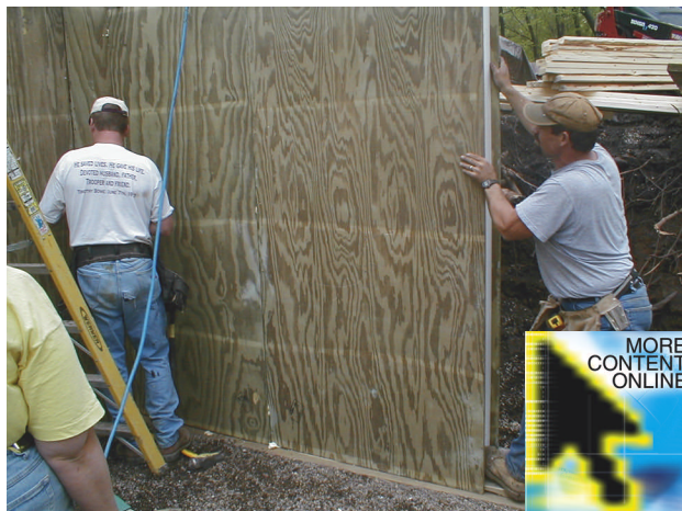
STRONG AND EFFICIENT SIPs designed for below-grade use can be installed by the same crew that will complete the structure.
